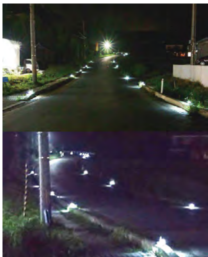
Fig. 6. Photos after the lighting arrangement of the escape route A.
